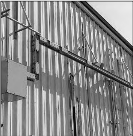
Complete outdoor run of Spectra Series busway.
