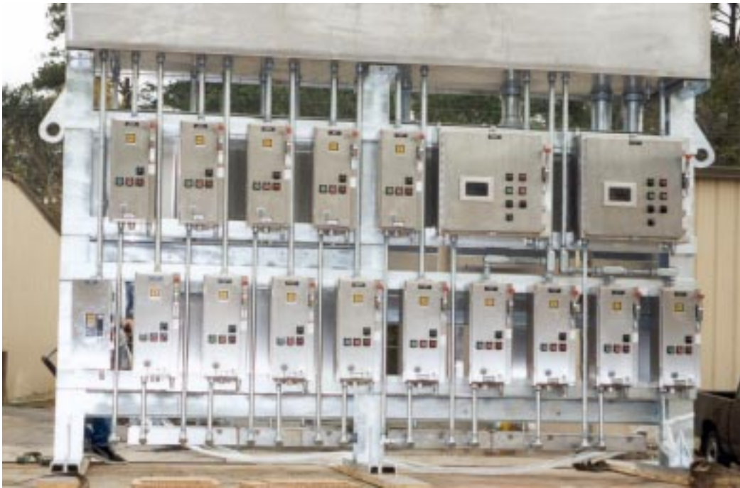
NEMA 4X stainless steel switchrack. The two units with windows are variable frequency drives.
